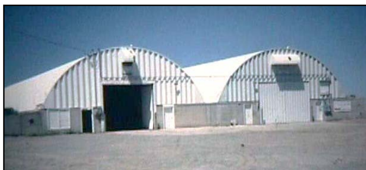
Figure 24. Modern potato storage facilities used to store potatoes in northern potato-production areas. Storage capacity can range from 500 ton to over 20,000 ton. Storage facilities are generally insulated and equipped with a forced-air ventilation system to control temperature and humidity. Most potatoes are stored in bulk piles, but box storages are utilized in some areas. (W. Bohl)
