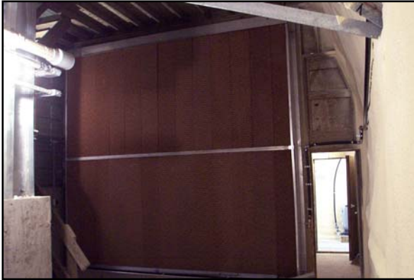
Figure 26. An evaporative cooling pad is constantly saturated with water while air is moved through the pad to provide humidity and cooling to potato tubers in storage. (S. Belyea)
